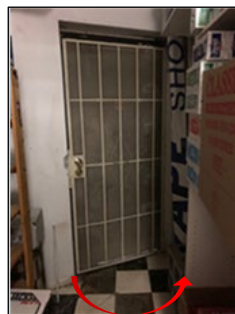
Chained with Lock
