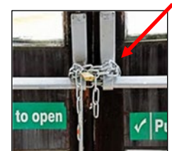
Chained with Lock IFC 1010.1.9
